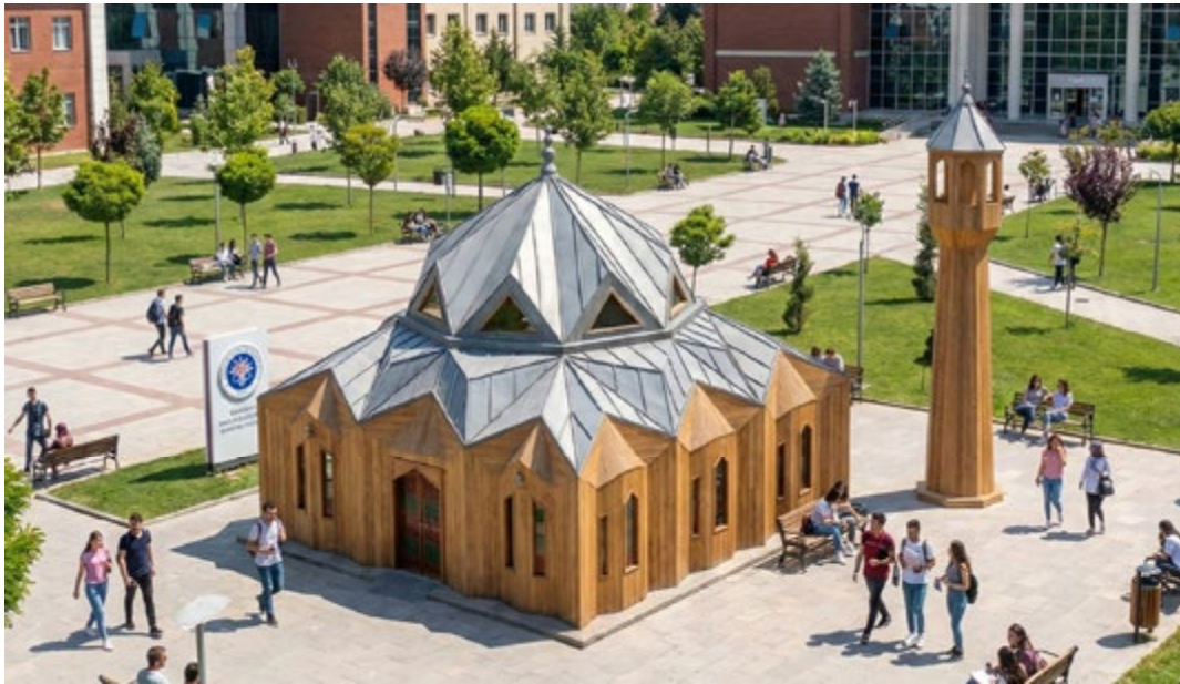
Figure 1: A representative visual of the morphological configuration of the Barkat timber folded plate construction system, organized according to the 6x6m-sized worship volume.
